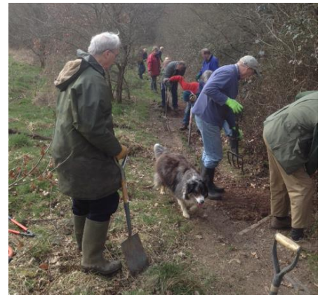
Volunteers hard at work repairing a path
